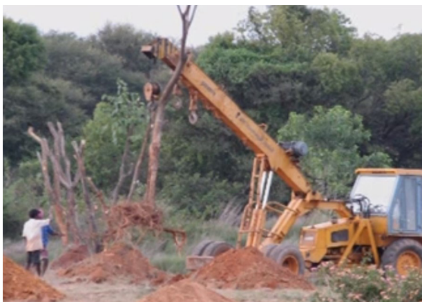
Clearing the site for construction; 2007.
