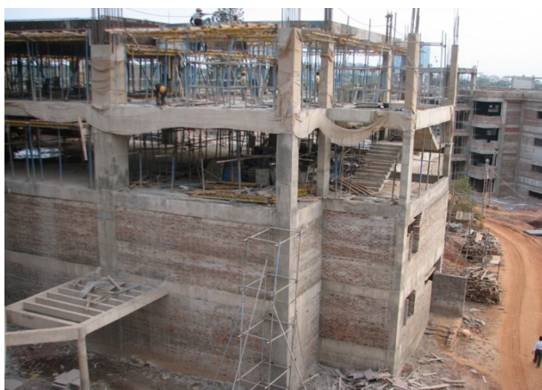
A flurry of construction activity; September 2009.
